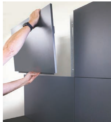
Back panels slot onto the backstrap system
